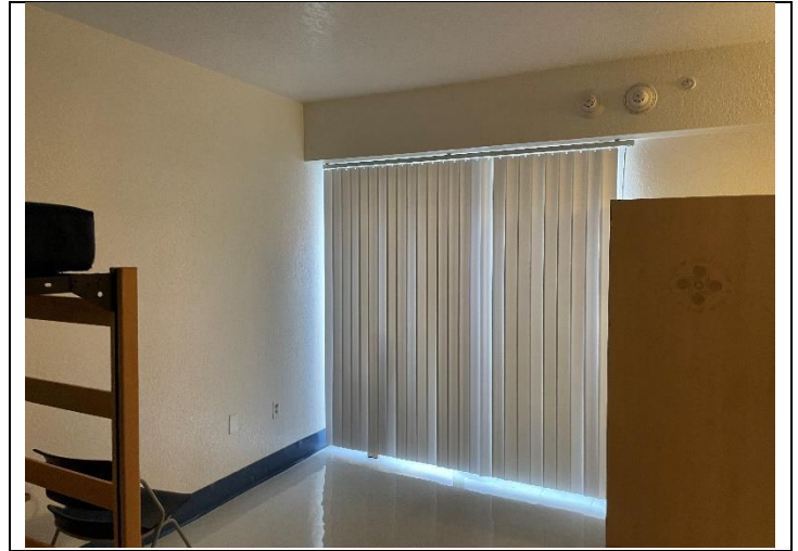
4. View of a typical PEI 2 unit (interior)
