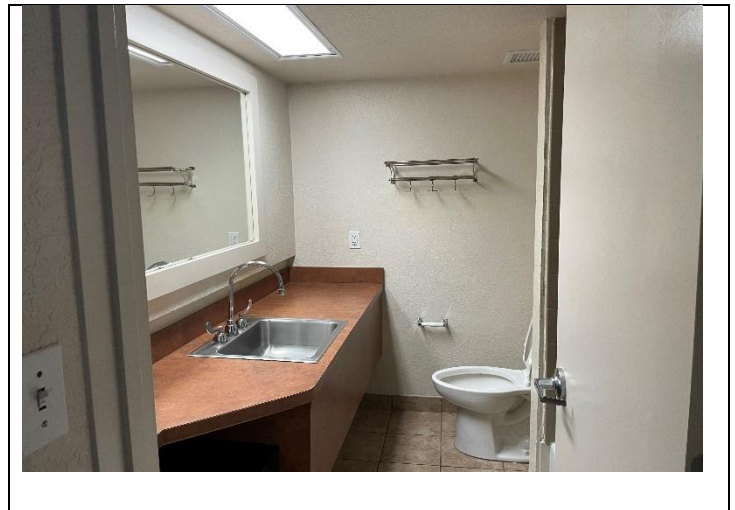
28. View of a typical PEI 3 unit restroom
