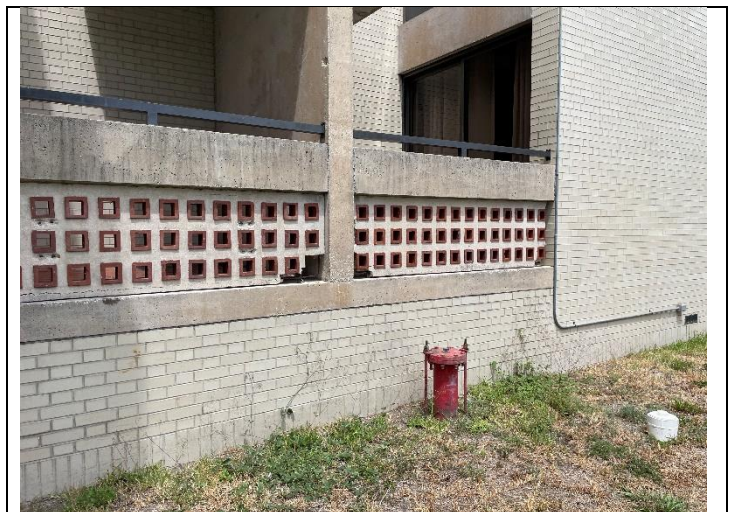
46. View of typical balcony for PEI 2 and 3 buildings with visible brick damage
