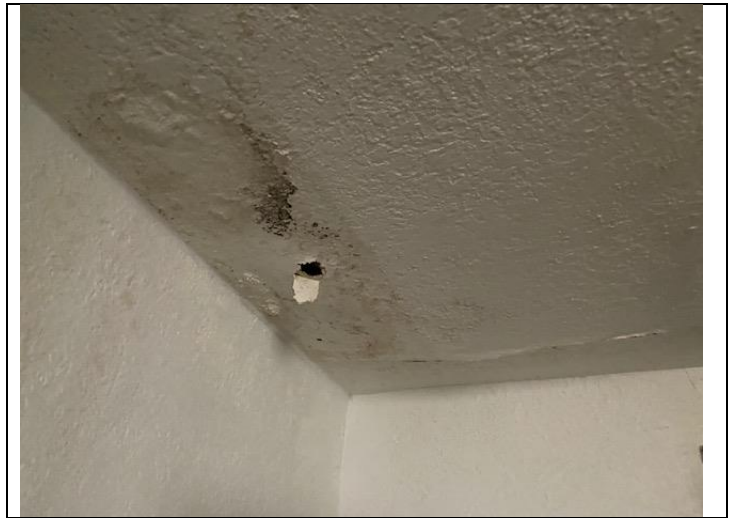
22. Close up view of SVG on ceiling outside restroom in PEI 2 Lounge
