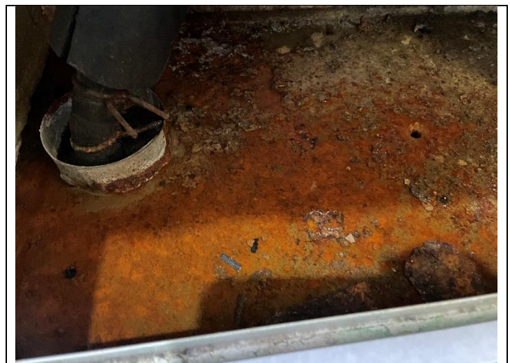
42. View of standing water in HVAC return box likely caused by drip pan out of alignment
