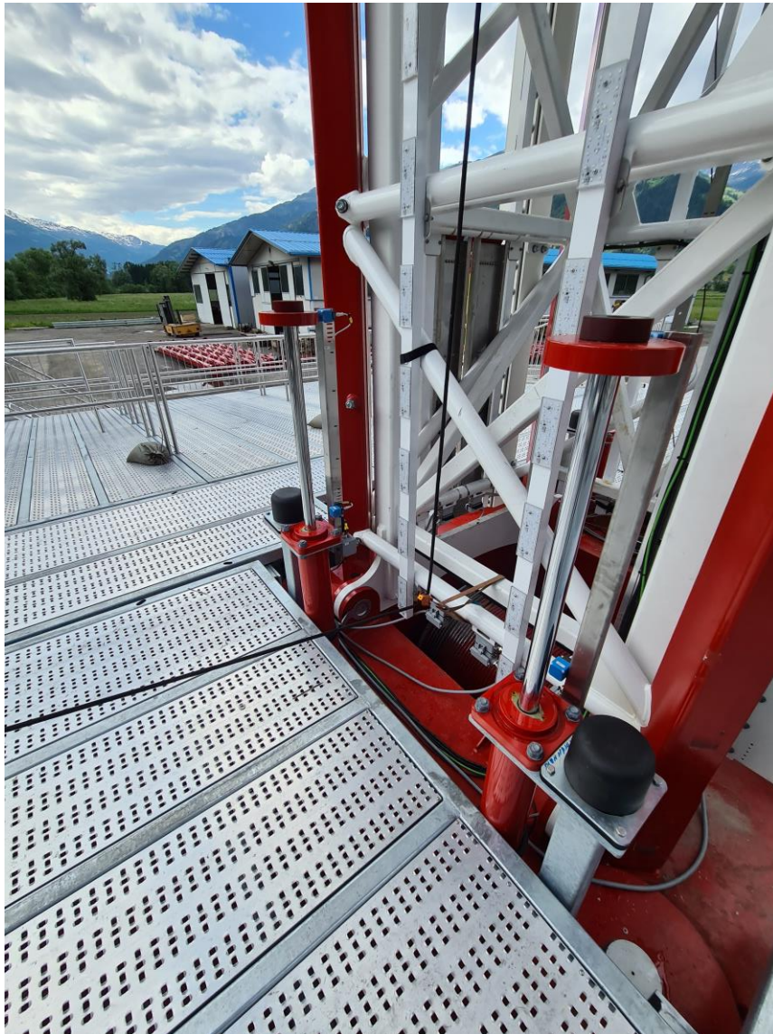
Figure 5-34 Pulley on the bottom side of tower
