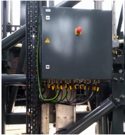
Figure2-5: Junction Box JB20
