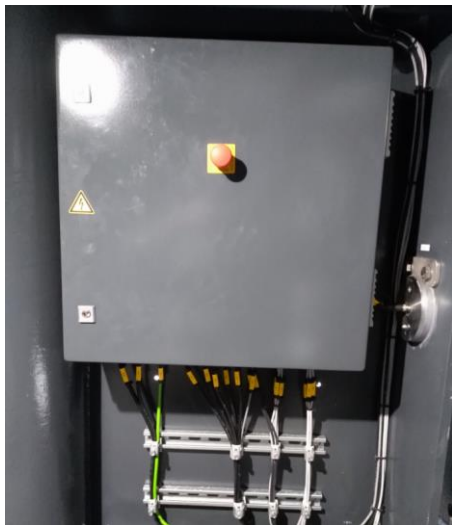
Figure2-6: Layout Junction Box JB40
